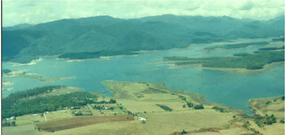
Plate 1: Aerial view of Pelican Point [centre of photo] looking from the western shore of Lake Tinaroo.
